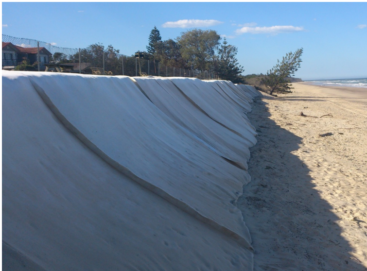
Photo 1 – Geotextile covering to limit wind erosion of embankment at Meridan Resort, Old Bar Beach (photo date 9/9/13)
