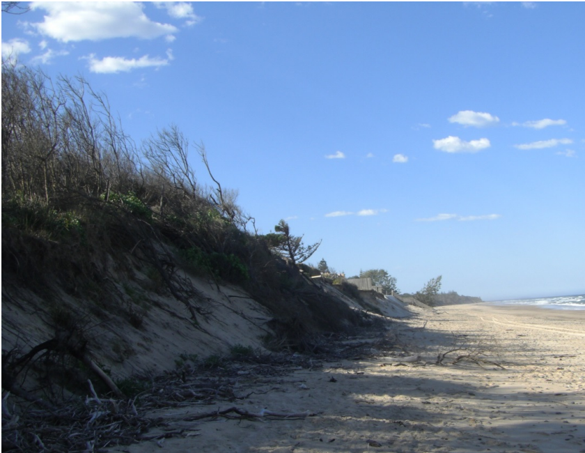
Photo 2 – Eroded dune at south end of Lewis Street subdivision (photo date 9/9/13)
